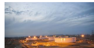
Tank Farms & Terminals
