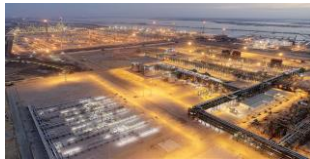
Gas Production Facilities & NGL Processes
